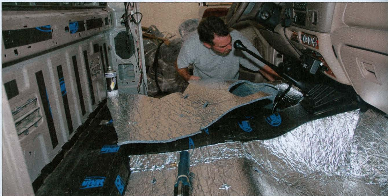
The entire floor and the rear cab wall were covered with the Heat Shield panels.
