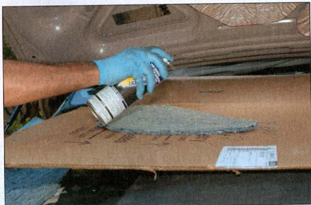
With the Dynamat in place, the panels of Acoustishield were installed using quick-dry spray contact glue.
