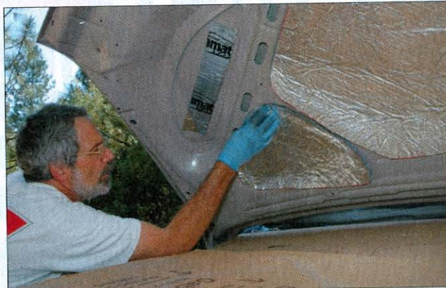
The Acoustishield panels were then pressed into position.
